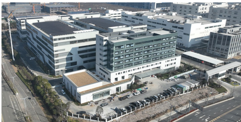
Installing Photovoltaic on the Rooftops of Sinexcel Suzhou
